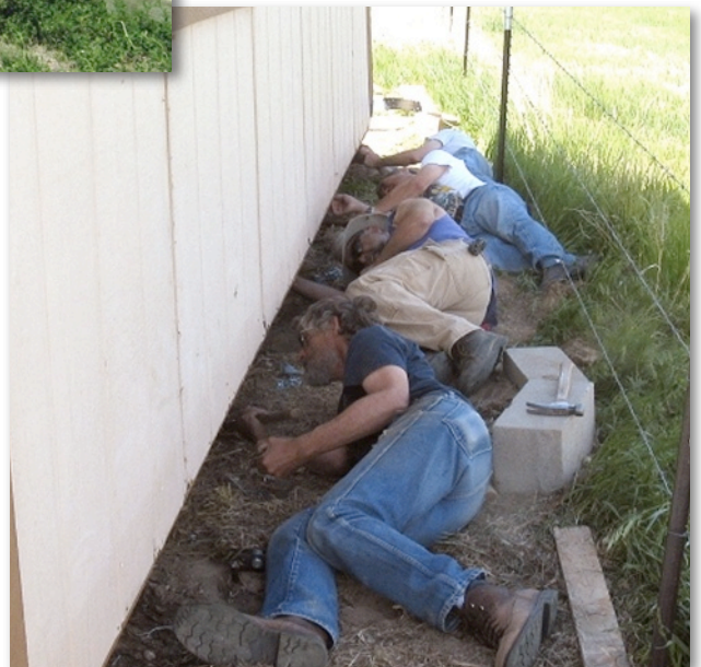
Above right, photo 4: Close work attaching hangers to a new 6x6 support timber, and below, photo 3: the warming hut is jacked up and ready for the installation of new support timber.
