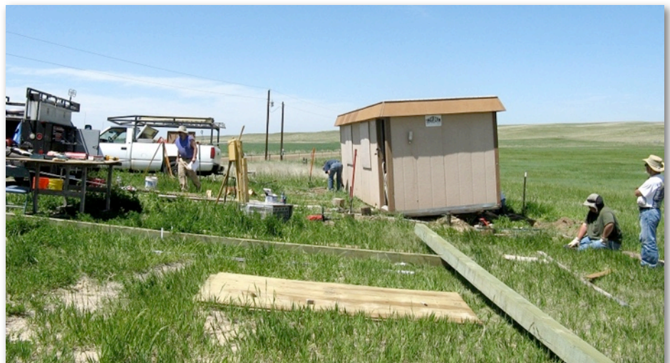
Above right, photo 4: Close work attaching hangers to a new 6x6 support timber, and below, photo 3: the warming hut is jacked up and ready for the installation of new support timber.
