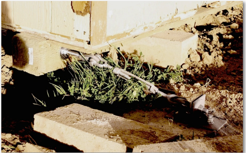
Photo 5: New improved anchor hardware.
